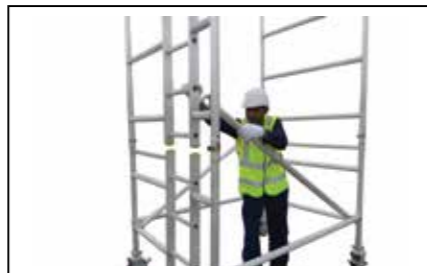
Step 7 Fit two diagonal braces yellow colour coded from the first rung of the structure, braces must be positioned in the opposite Direction as shown.
