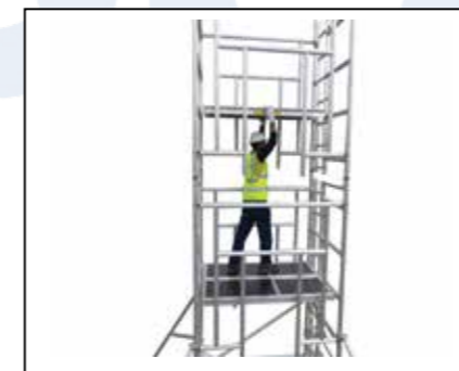
Step 13 Position platforms three rungs lower from the top and apply wind lock.
