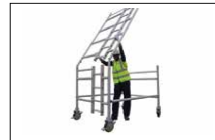
Step 5 Fit one span frame and one ladder frame to the lower frame. Make sure ladder frame is in one line.
