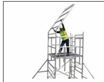
Step 11 Standing on the platform continue to build the structure following step 5,6, 8 & 9.
