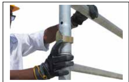
Step 6 After adding frames engage Interlocking clips.
