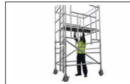
Step 9 Position one standard & one trapdoor three rungs lower from the top and apply wind lock (As ILLUSTRATION 3)
