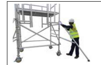
Step 10 Fit stabilisers ASAP to increase the base dimension .Position the stabilizer so that the foot pads are approximately equidistant from other at 45° for maximum stability.
