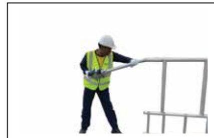
Step 2 Insert castor and adjustable leg in to the 2 rung span and ladder (or base frame) Make sure all the adjusting nuts are approximately at the same height.
