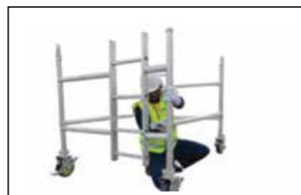
Step 3 Add two horizontal braces, blue colour coded to the bottom of the span frame and ladder frame rungs .Brace hook facing outside from the Inside.
