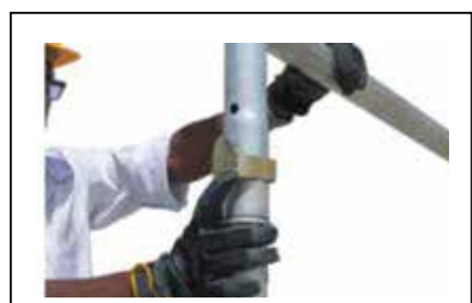
Step 6 After adding frames engage Interlocking clips.
