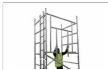
Step 8 Add advance guardrail frame to the top rung on both the sides.
