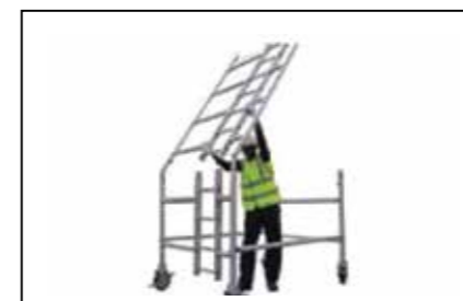
Step 5 Fit one span frame and one ladder frame to the lower frame. Make sure ladder frame is in one line.
