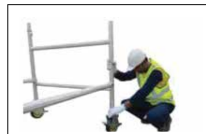
Step 4 Level the Mobile Tower . using spirit level. Use the adjustable jack of the wheel if require to level the tower
