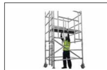
Step 9 Position one standard & one trapdoor three rungs lower from the top.Make sure trapdoor opening on the side of ladder frame. Apply wind lock. As Illustration3
