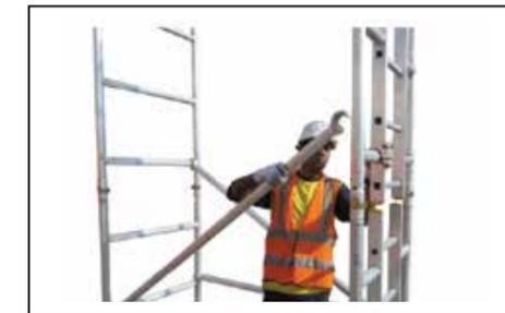
**Step 6** Position diagonal braces **YELLOW** colour coded From the first rung of both frame in a zig zag pattern from 1<sup>st</sup> to 3<sup>rd</sup> rung & 3<sup>rd</sup> to 5<sup>th</sup> rung either side of the tower opposing each other as illustrated Make sure diagonal brace is aligned.
