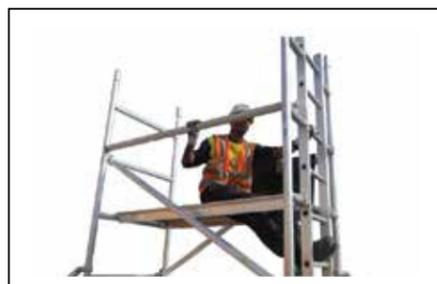
**Step 10** Sitting through the trapdoor add two horizontal braces on 5<sup>th</sup> & 6<sup>th</sup> rung ,two each on both end of the frame.
